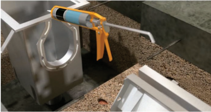
SILICON SEALANT APPLIED BETWEEN DRAIN FLANGE AND CATCH BASIN FLANGE
