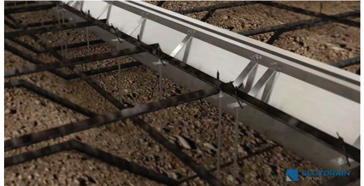
REBAR INSTALLATION BETWEEN THE FLOOR GRID AND THE LEVELING BAR
