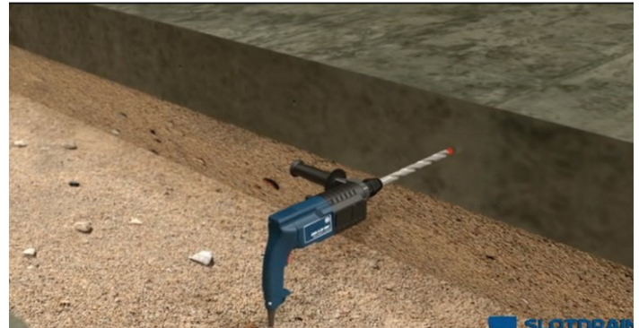
DRILL THE SIDES OF THE SLAB
