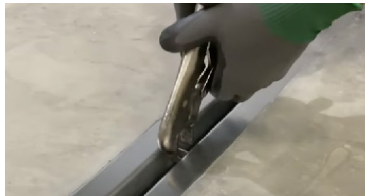
REMOVAL OF METAL TABS
