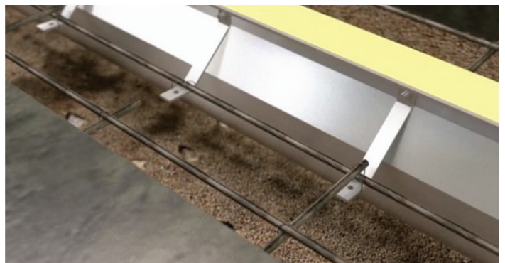
REBAR INSTALLATION BETWEEN THE DOWELS AND THE LEVELING BAR
