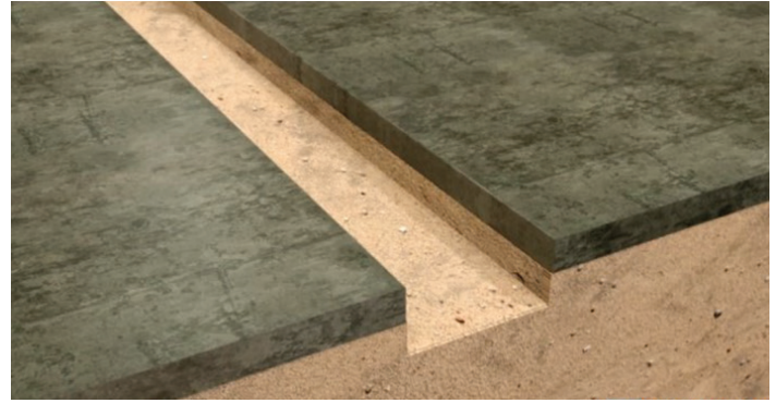
EXCAVATE THE TRENCH IN THE CUT SLAB LOCATION
